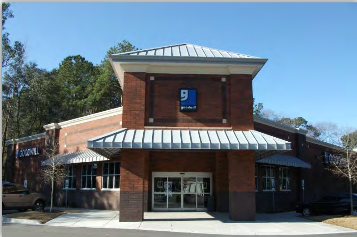
Goodwill Retail, Summerville (Old Trolley Rd), SC
